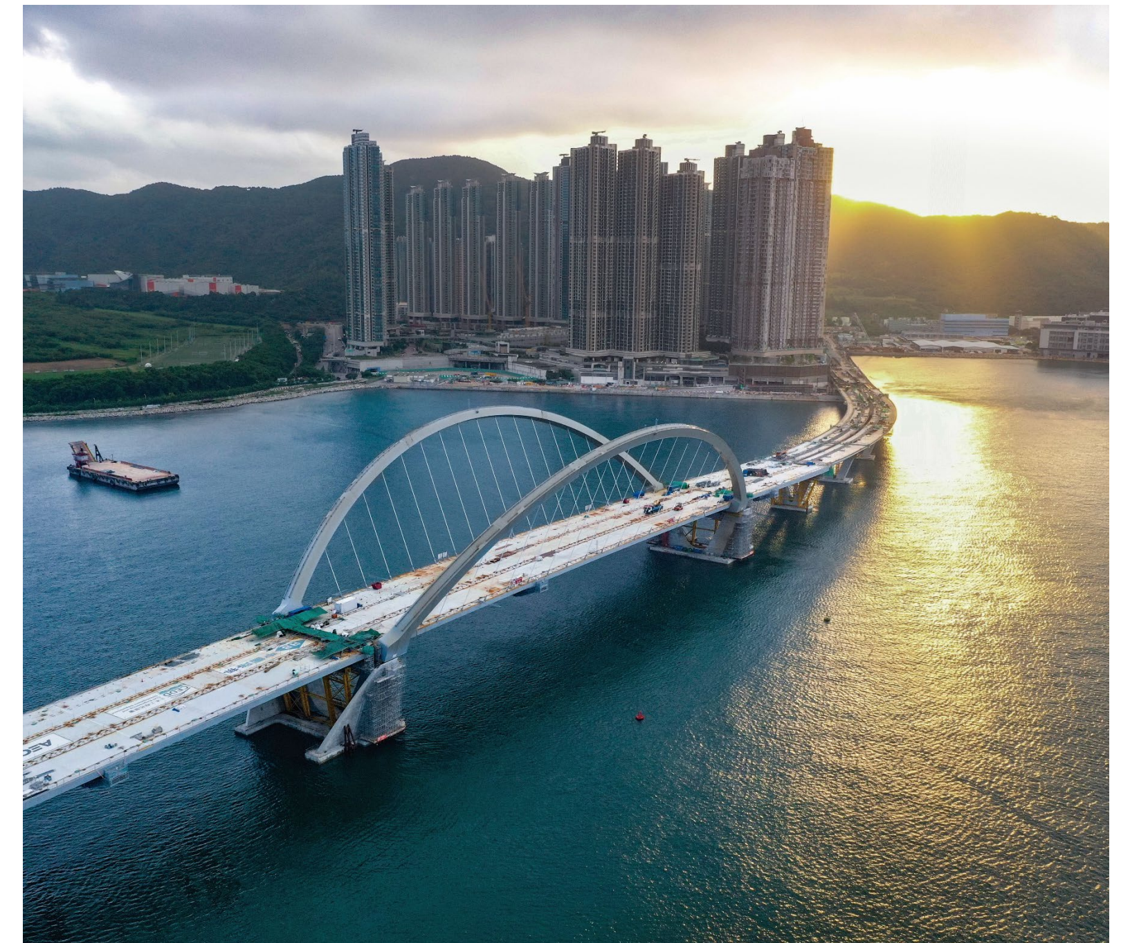
將軍澳 - 藍田隧道和將軍澳跨灣連接路 預計今年12月同步開通 TKO-Lam Tin Tunnel and Cross Bay Link, TKO Targeted commissioning in tandem in December this year
