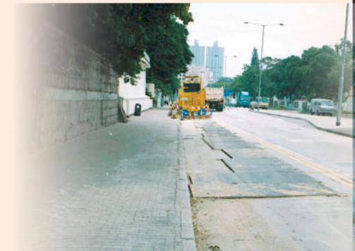
歌和老街行車線在道路工程施工時間以外鋪上鋼板，照常行車 The traffic lane at Cornwall Street covered by steel plates and open to traffic outside the working hours of the road works
