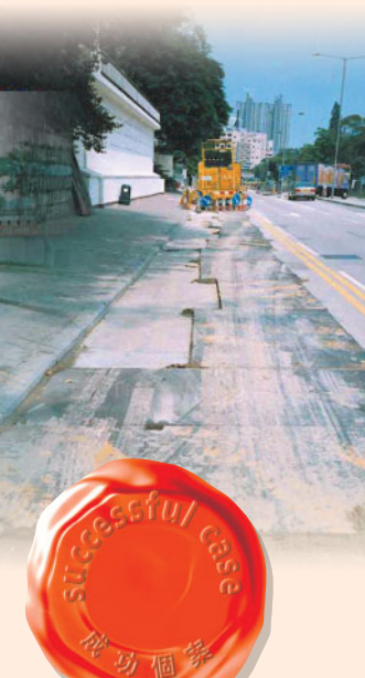
歌和老街行車線在道路工程施工時間以外鋪上鋼板，照常行車 The traffic lane at Cornwall Street covered by steel plates and open to traffic outside the working hours of the road works
